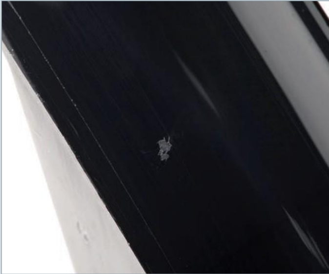
Surface blemish caused by a gate that has broken off (unreinforced Ultradur)
